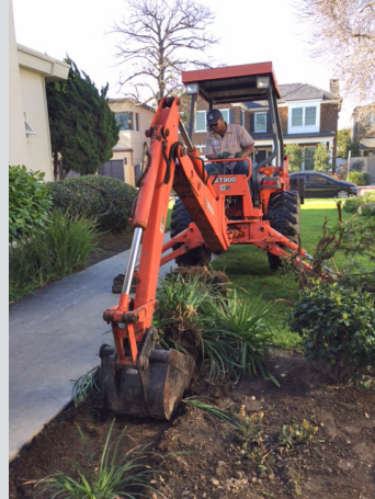
Skiploader removed thick roots.
