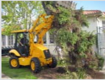
Large equipment needed.
